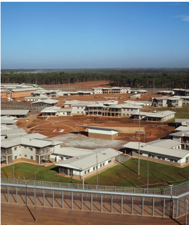
Darwin Correctional Precinct – Low security area at May 2014
